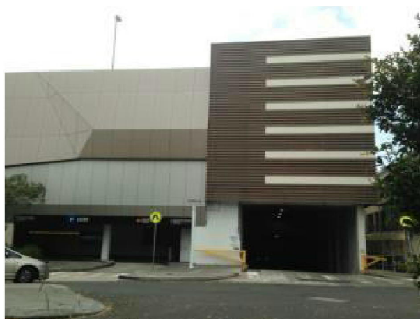
PICTURE 4 – EXISTING CAR PARK ENTRY ADJACENT TO 12-14 MALVERN AVENUE
