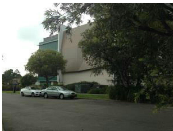
PICTURE 6 – LOOKING TOWARDS CORNER OF MALVERN AVENUE AND HAVILAH STREET.
