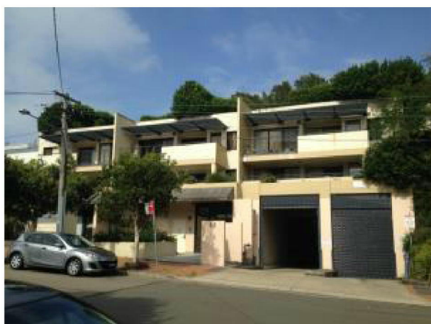
PICTURE 5 – EXISTING RESIDENTIAL FLAT BUILDING 3-5 HAVILAH STREET
