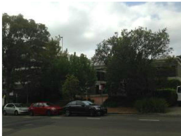
PICTURE 2 – EXISTING BUILDING 12-14 MALVERN AVE
